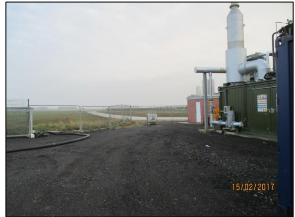
View of site (looking north)
